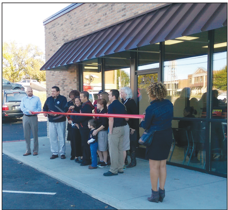
Little Caesar's Pizza, totally destroyed by fire last year, had its grand reopening on Monday, October 26th. It is located at 220 North Florissant Road. The store had to be rebuilt from the ground up. Hidden Treasures, an antique store also housed in the building will be open again soon.
