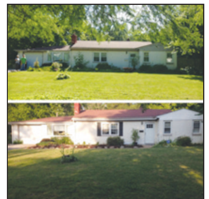
The Vaz-Fisher home, before (top), and after (bottom) the curb appeal day.
