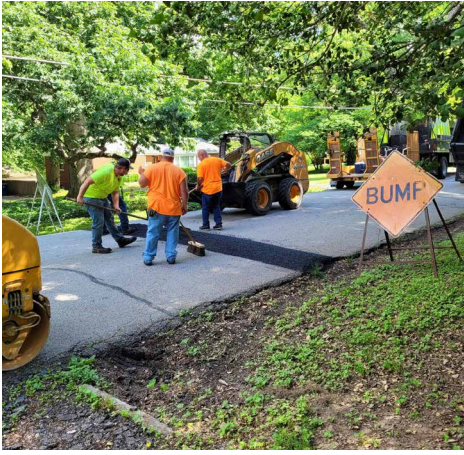
Crews installing speed bumps along Calverton Road
