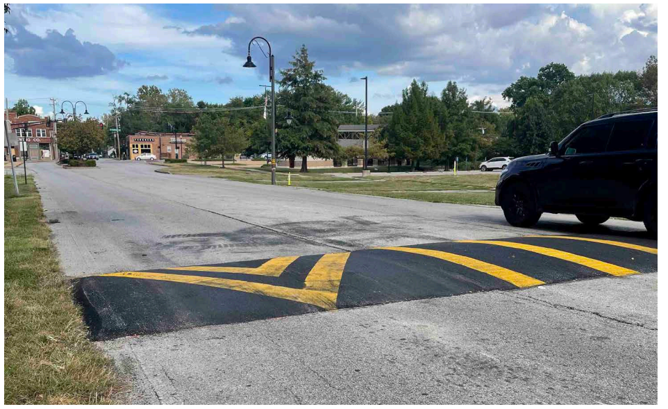
This speed hump, near the Ferguson Farmer’s Market is one of six recently installed on Dade.
